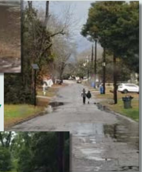
Street in Scottsville flooded due to poor drainage
