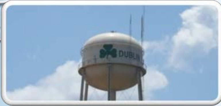
ELM STREET TANK 250,000
